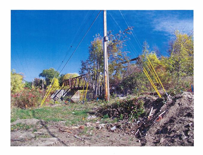
Figure 2 Concord Pole 50 on south side of Merrimack River showing recently installed guying to support increased tensions applied to pole resulting from aerial crossing.
