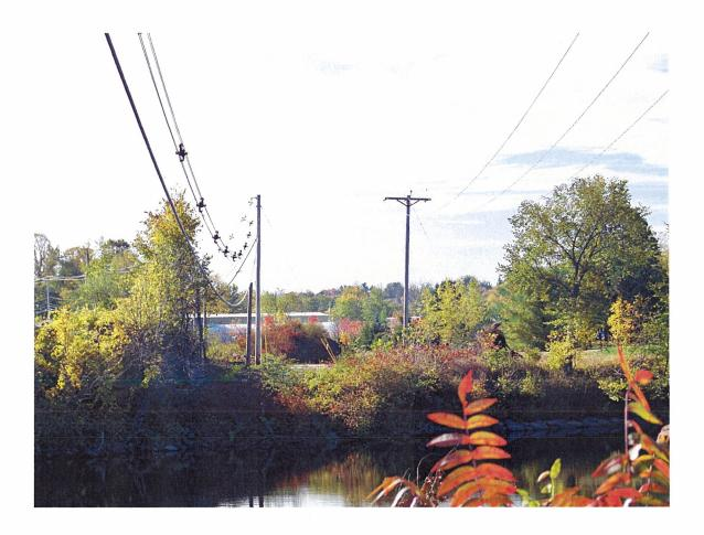
Figure 1 Merrimack River Crossing looking southerly. Aerial Cable Crossing and Electric Crossing are shown on the Left and are subject to this license. Unitil 34.5kv crossing is shown on the right and is not the subject of this license.
